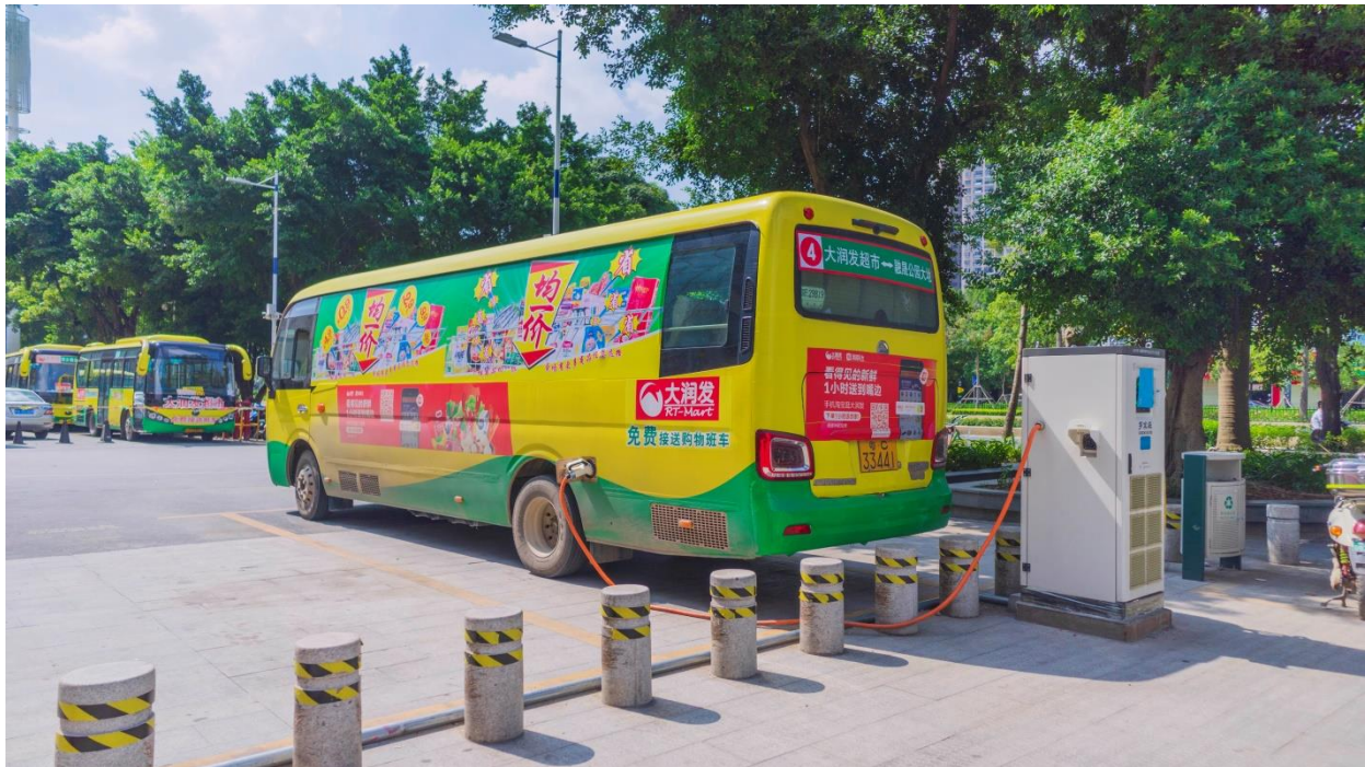
An electric bus at a charging station. Source: Mars Hartdegen/Flickr
