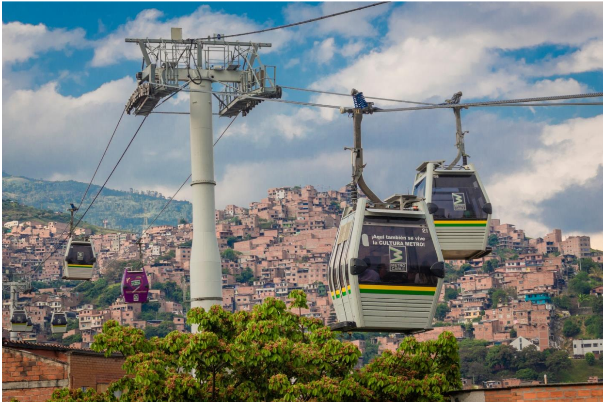
Cable cars along the Metrocable Line J of the Medellín Metro. Source: Alexander Canas Arango/Shutterstock
