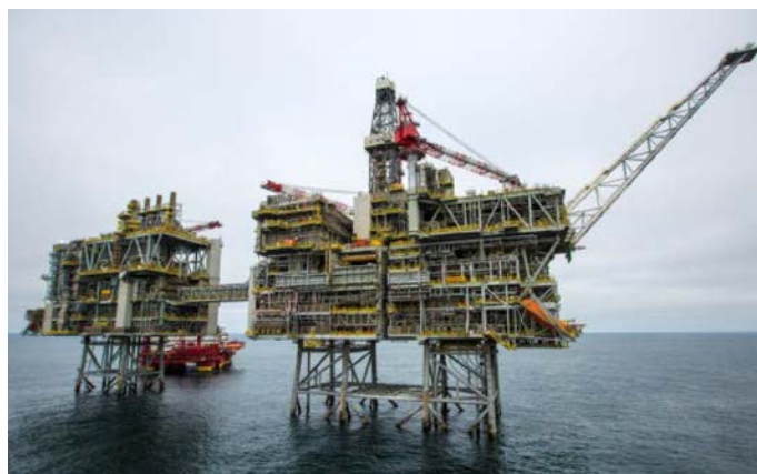
Figure 1: The Clair Ridge DP and QU platforms
