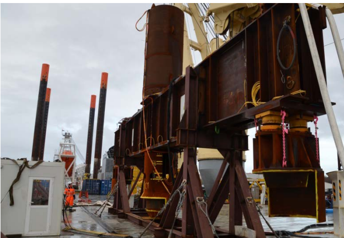
Figure 6: Load test beam and frame
