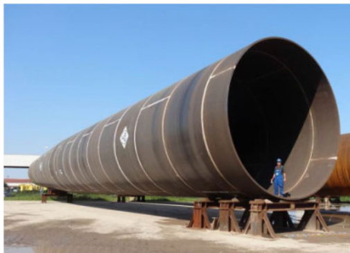
Figure 1. Monopile for Gode Wind offshore wind farm (diameter = 7.5 m at seabed).
